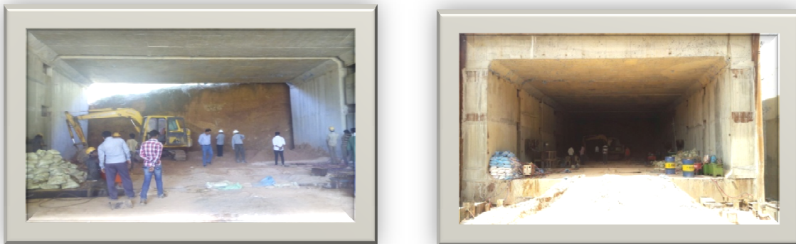
Figure 3: Box Pushing Operation under Progress
